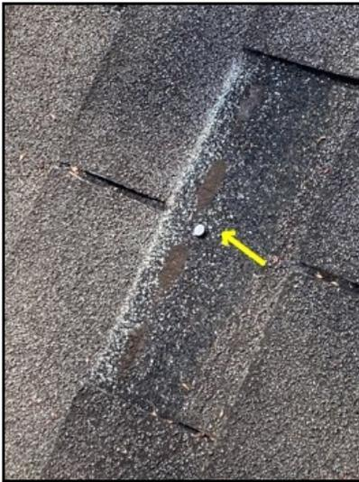
Missing shingle and exposed nail head.
