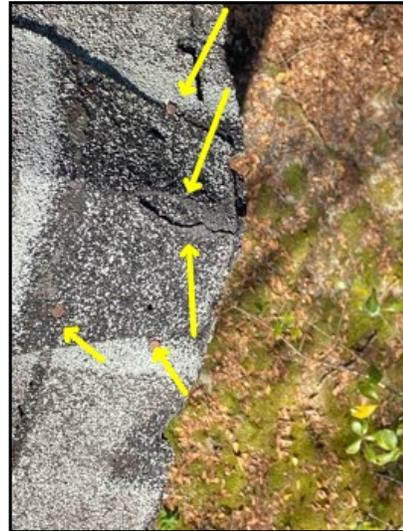
Damaged shingle and exposed nails
