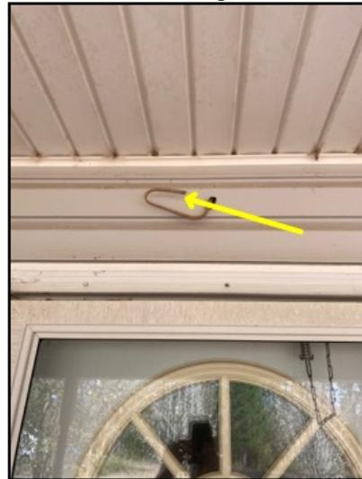
Exposed electrical wiring on the front porch
