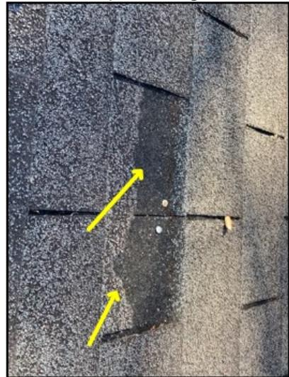
Missing shingle and exposed nail
